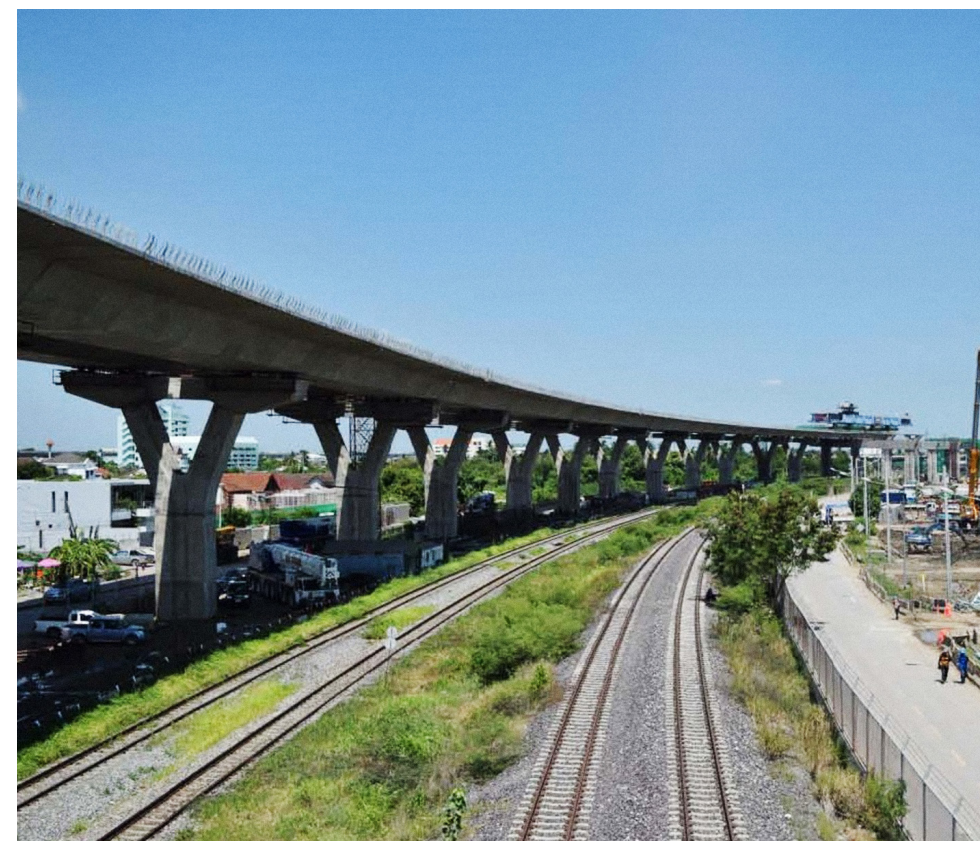
◀ SRI RAT-EXPRESSWAY STAGE 3/5 RENOVATION
