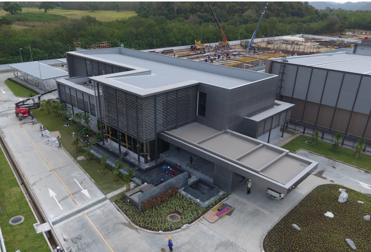
▼ INET DATA CENTER 3, SARABURI
